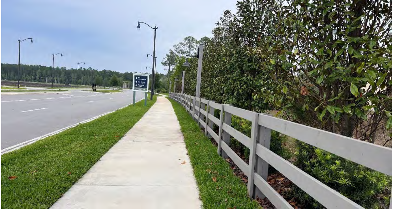
Sidewalk and Fencing Along everRange Entrance
